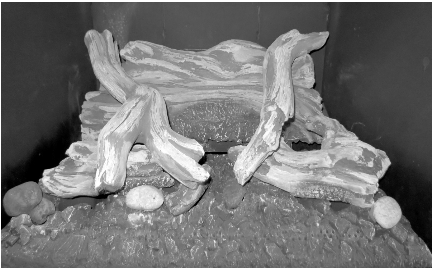
Figure 7.36. Beach Fire Final assembly. Use a toothbrush or tweezers to lightly disburse small tufts of ember fibers across the front of the burner base.
